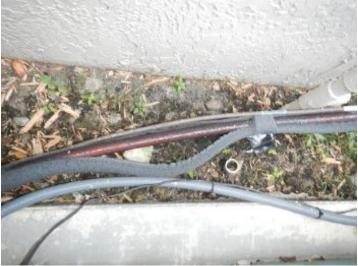
LOWSIDE INSULATION:. Low side line coming out of the condenser unit needs to be re-insulated.
