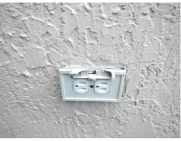
GFCI's:, Outlet cover is broken and not waterproof. Replace.
