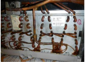
No excess signs of corrosion on your HVAC coils. This is what we look at to determine if there may be Chinese Drywall present in the home. Although this method cannot completely rule out the presence of Chinese Drywall it's a good indication that this home doesn't have enough to warrant any extra testing measures.
