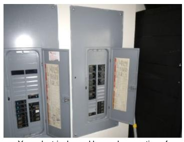
Your electrical panel has a demarcation of breakers and where those breakers are located. When working on the electrical inside the home it should be performed by a licensed electrician and the demarcation should not be relied upon as fact. Lack of power to the component that is being worked on should always be confirmed with an electrical meter.
