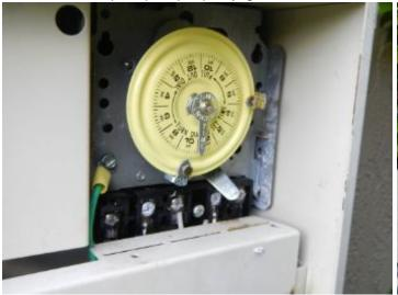
POOL TIMER:, Timer operated the pool pump/motor by the on/off switch at the time of inspection. The timing functions were not checked due to time constraints.
