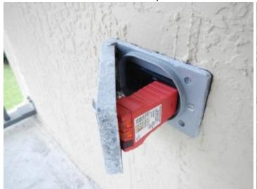
GFCI trip test failed on balcony outlet. Recommend replacing it.
