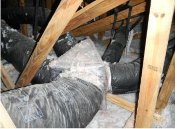
HVAC DUCTS:, No major system safety or function concerns with visible HVAC ducts noted at time of inspection. Minor hole noted in one of the HVAC ducts. Tape it up.
