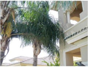
Tree branches overhanging roof and/or against siding. Trim trees that are in contact or proximity to home, as branches can abrade siding and damage roofing.
