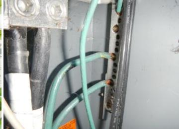
Proper ground for your exterior electrical panel is noted.
