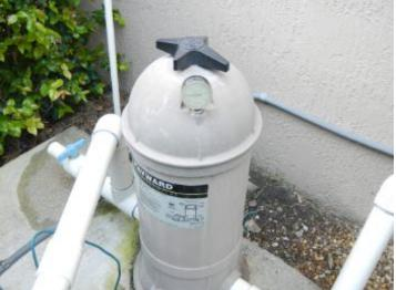
POOL FILTER:, Unable to determine the the condition of the pool filter. The Bullet type filter was unable to be opened with reasonable force. Have this checked and repaired by a licensed pool company.
