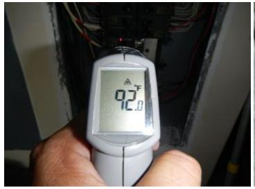
Your electrical panel was checked for proper grounding, loose connections, overheating and double tapped beakers. None were found at the time of inspection.
