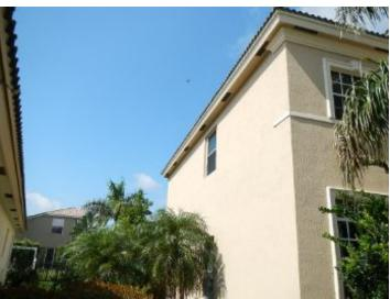
No gutters or downspouts. Full installation recommended to keep water away from structure. Water can weaken the foundation and deteriorate the siding. Be sure to install splashblocks or extensions to carry water away, and keep water from areas such as driveways or walks where it can be a slip hazard during rainy season.
