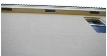
VENTS:, No major system safety or function concerns with attic venting noted at time of inspection., Soffit vents noted.
