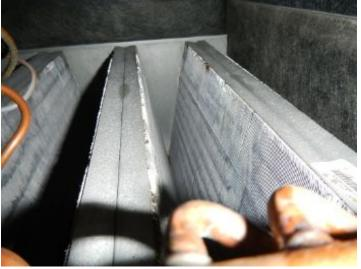
HVAC COILS:, HVAC Coils need to be cleaned. Organic growth noted under the evaporator coils. Make sure to have the technician clean these areas in both air handlers at the time of service. This could become an irritant such as itchy eyes, runny noses or even a health hazard such as strep, staff infection or even Legionnaires Disease.
