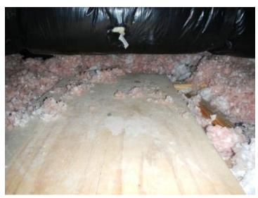
HATCH:, Maintenance Tip: Keep attic hatch sealed/caulked to minimize warm moist air escaping to attic during the winter and cool air in the summer, which could promote conditions conducive to mold growth. It should also be insulated to increase energy efficiency.
