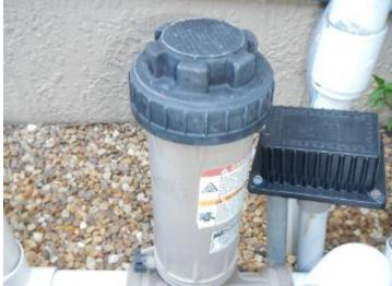
Automatic chlorine feeder was operating at the time of inspection.
