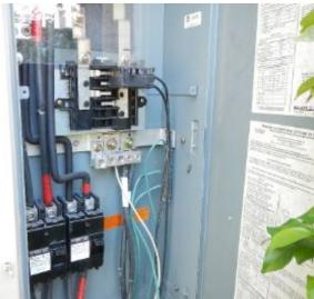
EXTERIOR MAIN ELECTRICAL PANEL:, Your exterior main electrical panel was checked for proper grounding, rust and corrosion.
