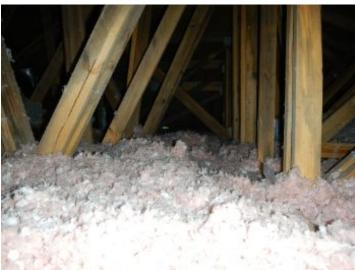
INSULATION:, Cellulose Insulation noted., Insulation averages about 8-10 inches in depth
