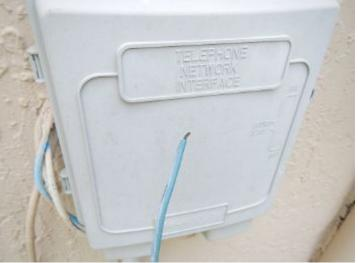
TELEPHONE SYSTEM: , Your telephone system is not properly grounded.
