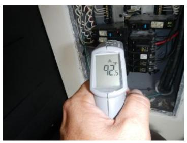
Your electrical panel was checked for proper grounding, loose connections, overheating and double tapped beakers. None were found at the time of inspection.
