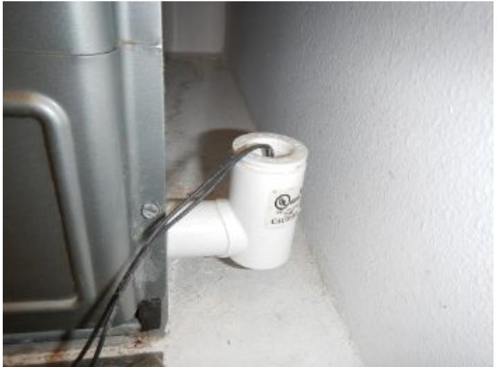
CONDENSATE LINE: Your HVAC system is equipped with a float switch which detects water backing up from the condensate line. If water does backup from the condensate line into the drain pan this switch will deactivate the entire HVAC system as not to allow water to overflow into the residence.
