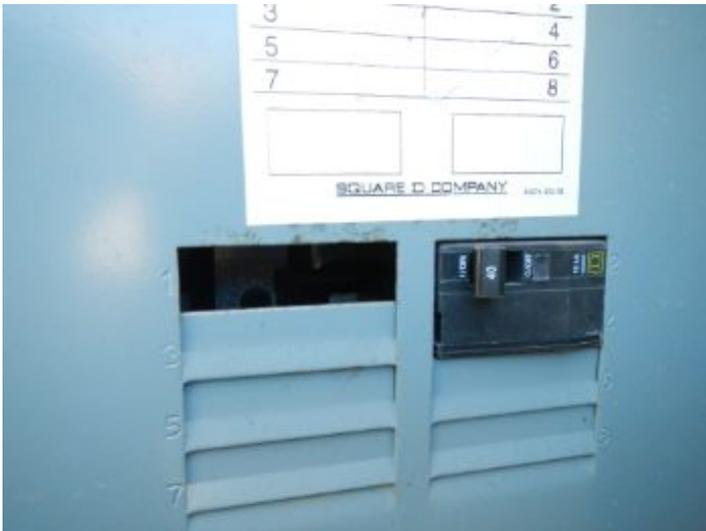
Missing cover blank on exterior service panel. Recommend replacing this to prevent electrical hazard.
