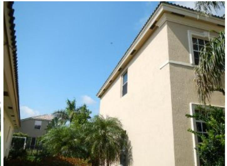
No gutters or downspouts. Full installation recommended to keep water away from structure. Water can weaken the foundation and deteriorate the siding. Be sure to install splashblocks or extensions to carry water away, and keep water from areas such as driveways or walks where it can be a slip hazard during rainy season.
