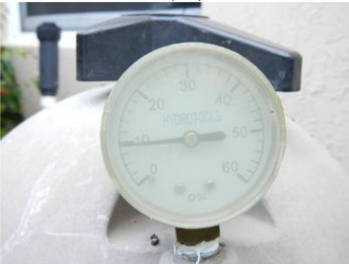
**BACKPRESSURE GAUGE:**, 10 PSI at the time of inspection. Anything over 20 PSI, it's time to clean the filter.
