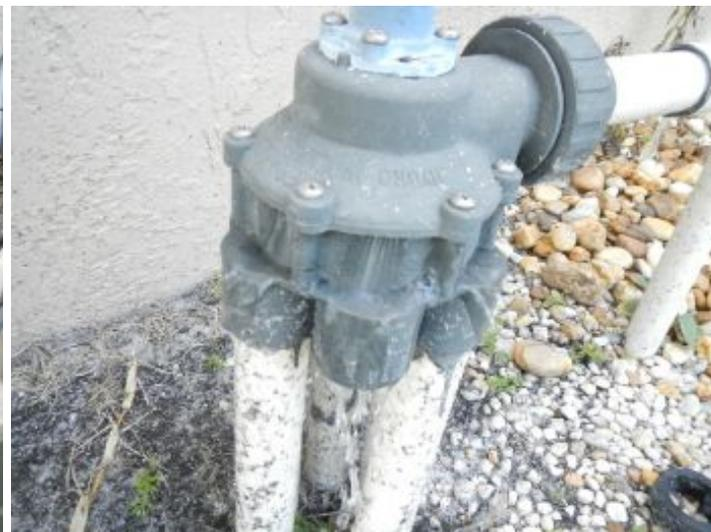
Main water shut off valve for the interior plumbing. IRRIGATION: Replace seals in the main irrigation valve.
