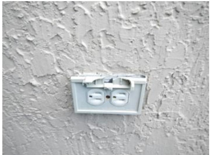
GFCI's, Outlet cover is broken and not waterproof. Replace.
