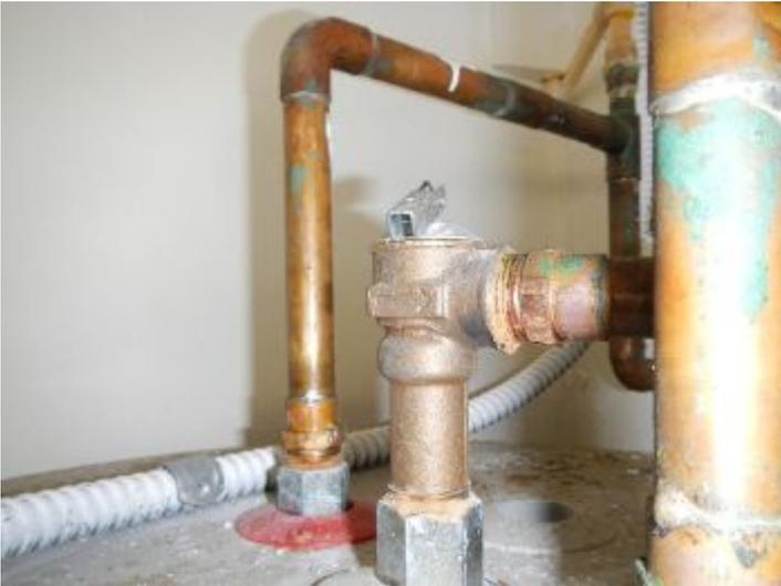
Temporary pressure relief valve was tested and operated properly at the time of inspection.
